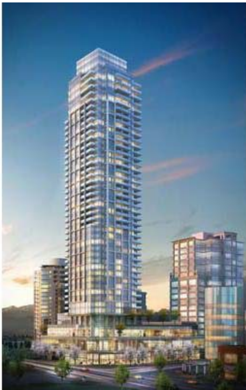
Sovereign, Burnaby's tallest highrise at more than 500 feet, is slated for completion in the spring of 2014.
